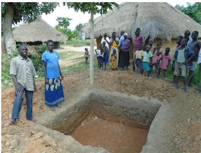
Newly constructed Rubbish (Refuse) Pit – IRT step up
