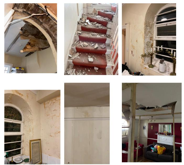
Some pictures to give you an idea of how things are in the Presbytery! From top: part of a door frame which crashed last year; the bottom pictures show some places where the water is leaking through the walls and walls with deep water ingress. The last picture is the hole in the roof we've been working on the last five months. Just some of the work that needs doing!
