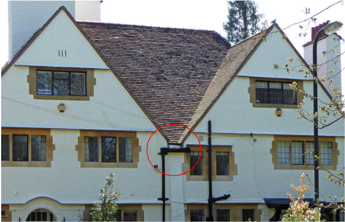
A larger version of the same crenellated rainwater head at Hollybank (1903)
