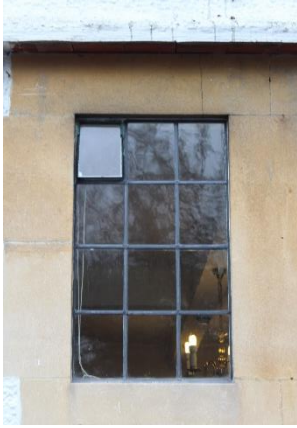
Single-opening pane visible in the top left
